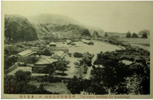
Fig. 1. Burnt island detention centre for vagrants.
