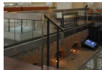
Fig. 7. In situ display of the raised foundation in the former Tainan prefecture hall.
